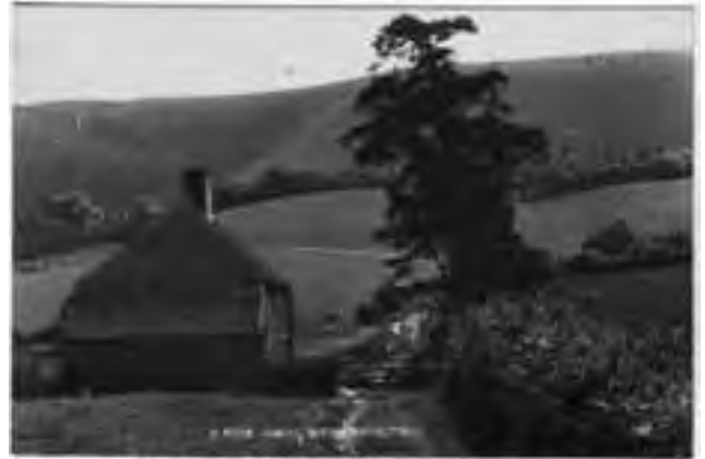
Above: Coldharbour, Greyfriars Lane, Storrington.
