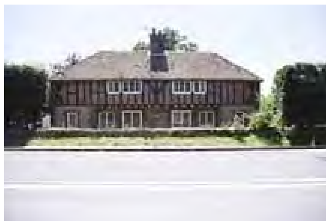
Chanctonbury Lodge, Storrington Road, Sullington (above). Restored C17 or earlier timber-framed building with modern red brick infilling.
