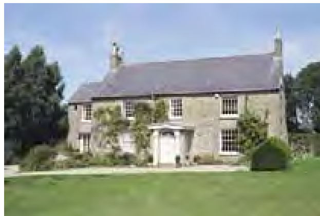
Hurston Place Farmhouse, Hurston Lane, Storrington (above).
